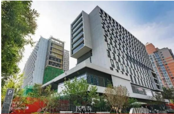
Beijing - Port Apartment | Yuan Er - Chengshousi Community
