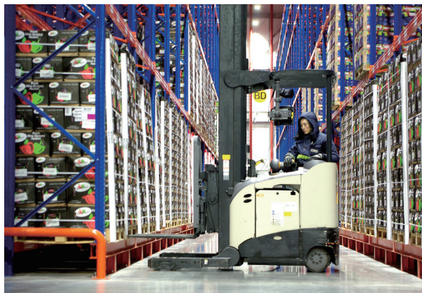
• VX Shanghai Haigang Cold Chain Logistics Park
