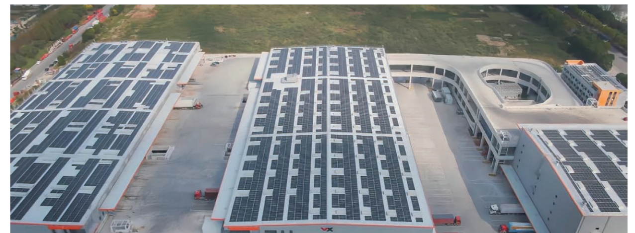
PV Distributed Power Station in VX Shanghai Fengxian Lingang Park
