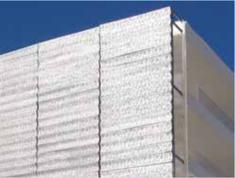
闭合固定百叶窗玻璃结构 Louvre Design I: Fixed closed louver with structural glazing
