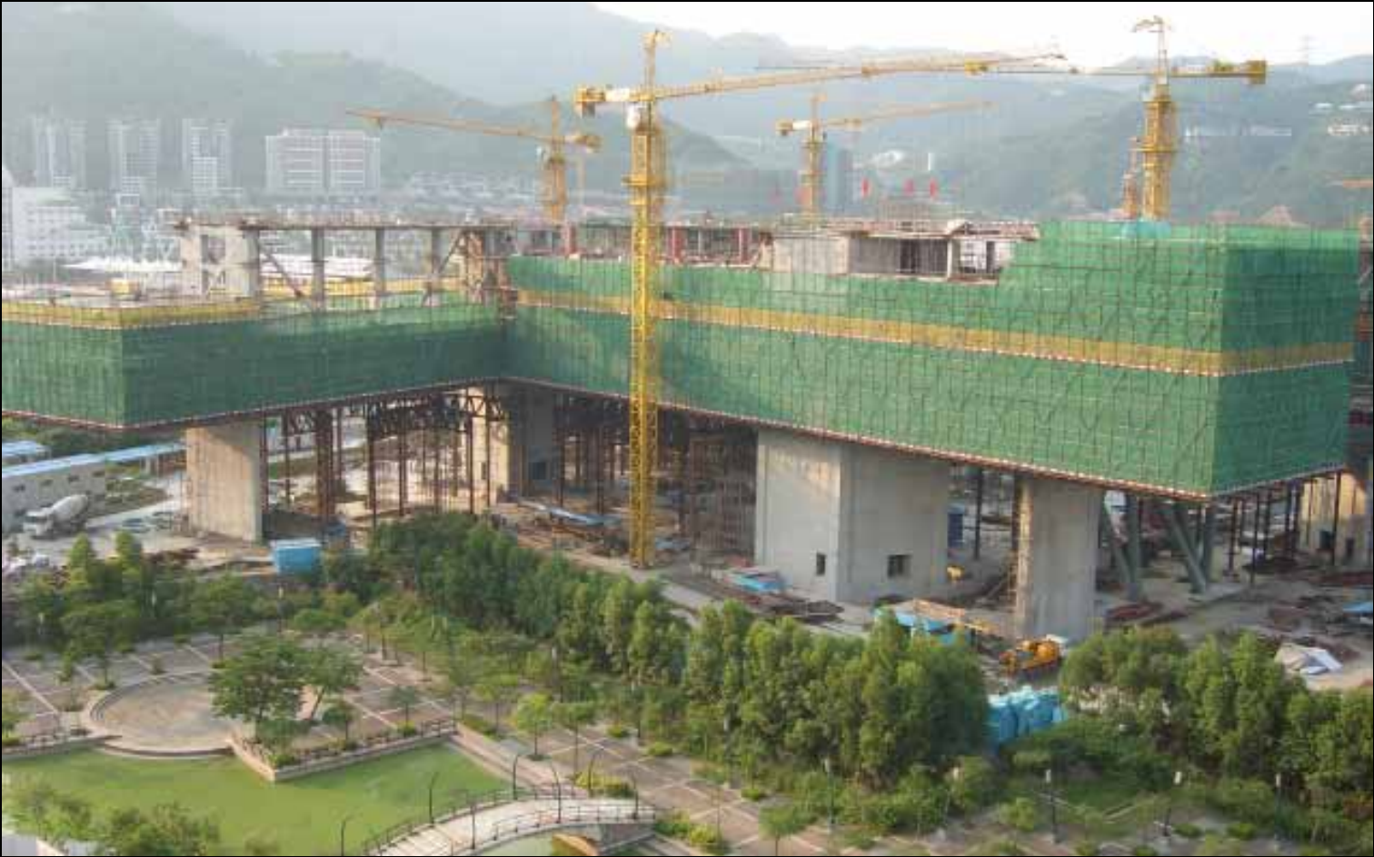
2008年3月, 上部结构逆作法。 March 2008, Reverse construction method was carried out.
