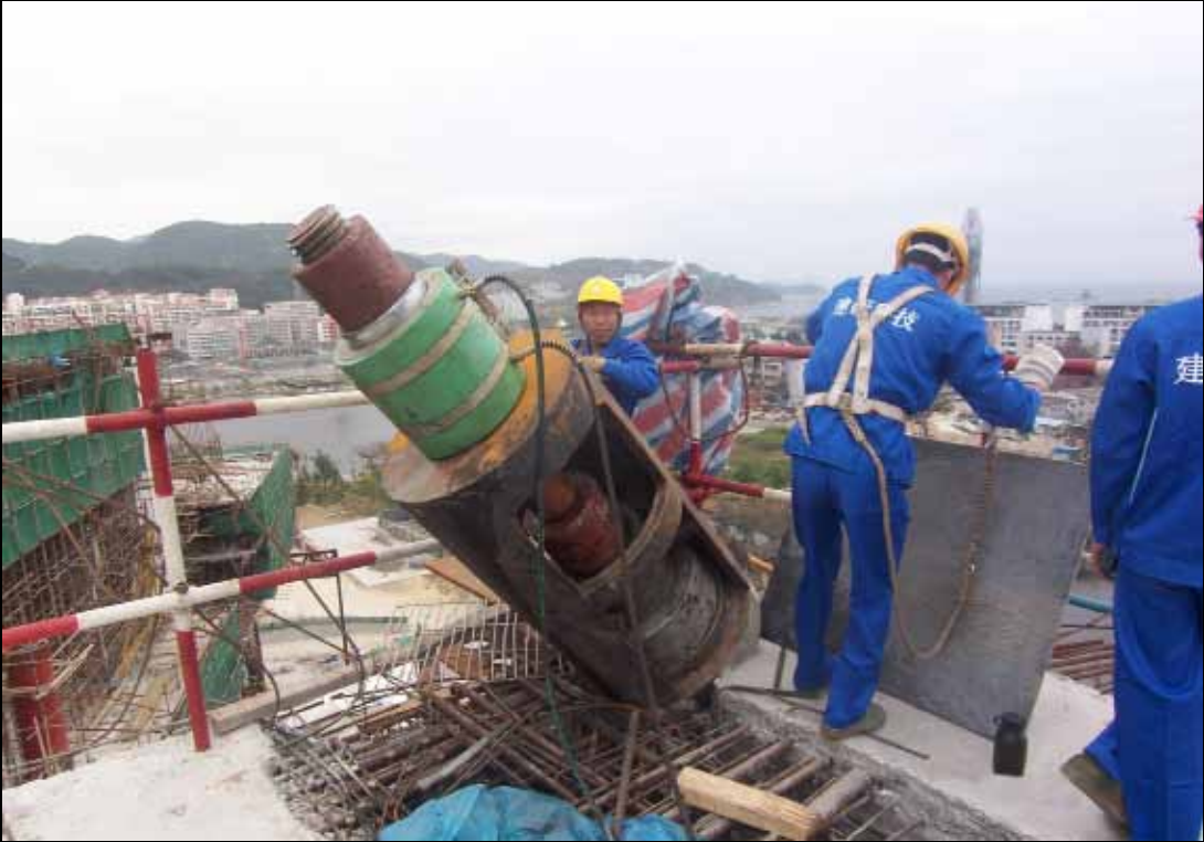
首次张拉中, 施工人员用千斤顶拉紧拉索。 December 2008, the lifting jack is straining cables.
