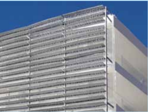
开启固定百叶窗玻璃结构 Louvre Design II: Fixed open louver with structural glazing
